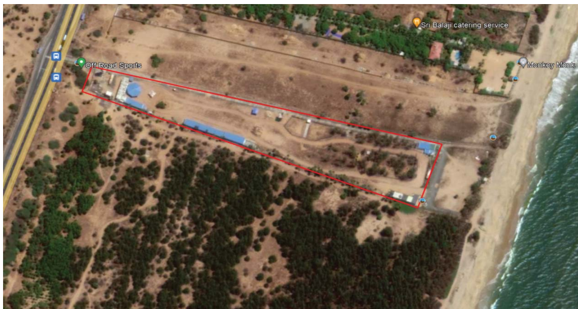
Fig. 8: Satellite image (March 2021) of racetrack constructed in CRZ 1A and NDZ area
