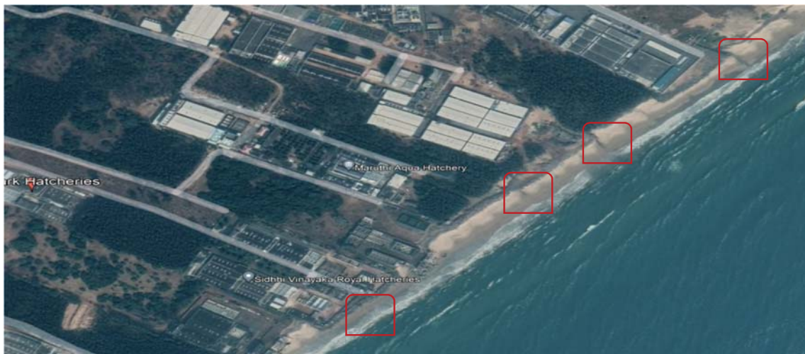
Fig. 18: Presence of many hatcheries on coastline and open discharge of the effluent into sea by hatcheries on Konapapapeta beach, East Godavari district.
